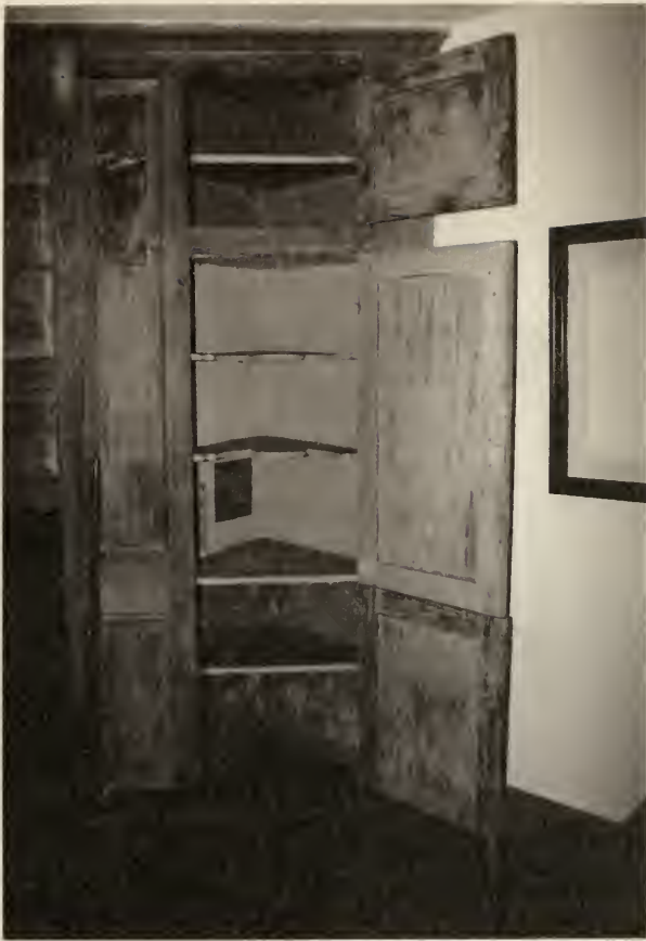
Figure 12. Detail of cabinet in second floor northeast room, fireplace wall paneling. (1993)
